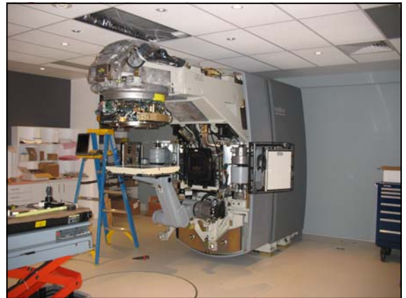
A Linear Accelerator being commissioned in Bunker 5
